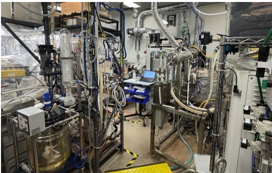
Figure 4: Pilot plant setup at the Boucherville facility
